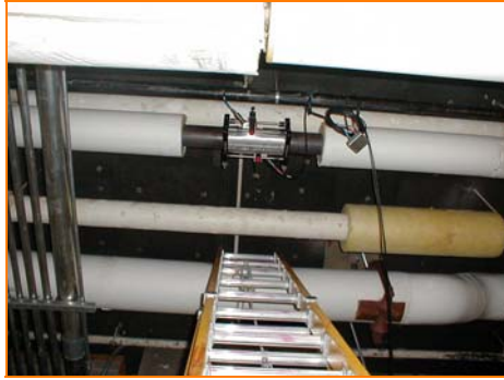
Figure 1: Clamp-on steam installation on a 4-inch line at Christie
